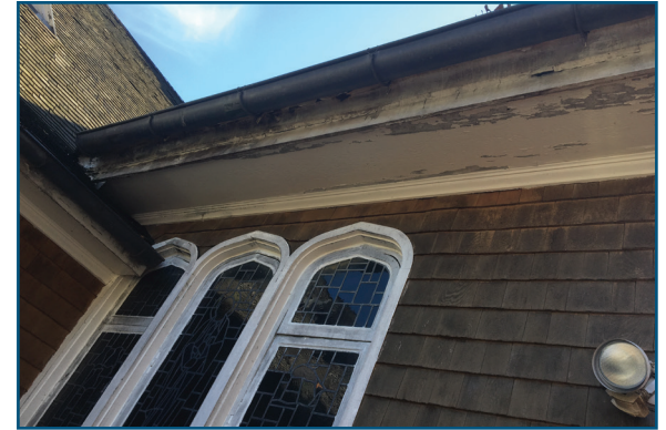
The window frames and trim will be repaired and painted
